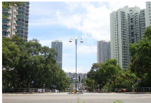
LR7 Road and Urban Infrastructure
